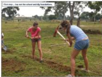
First step... Lay out the school and dig foundations.
